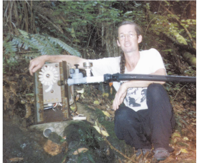
Above: Neale Blaymire's hydro system.
